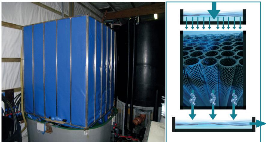
*Figure 2.13 Photo and drawing of trickling filter wrapped in a blue plastic liner to eliminate splashing on the floor (Billund Akvakulturservice, Denmark). The aeration/stripping process is also called CO<sub>2</sub>-stripping. The media in the trickling filter typically consists of the same type of media as used in fixed bed biofilters – see figure 2.10.*
